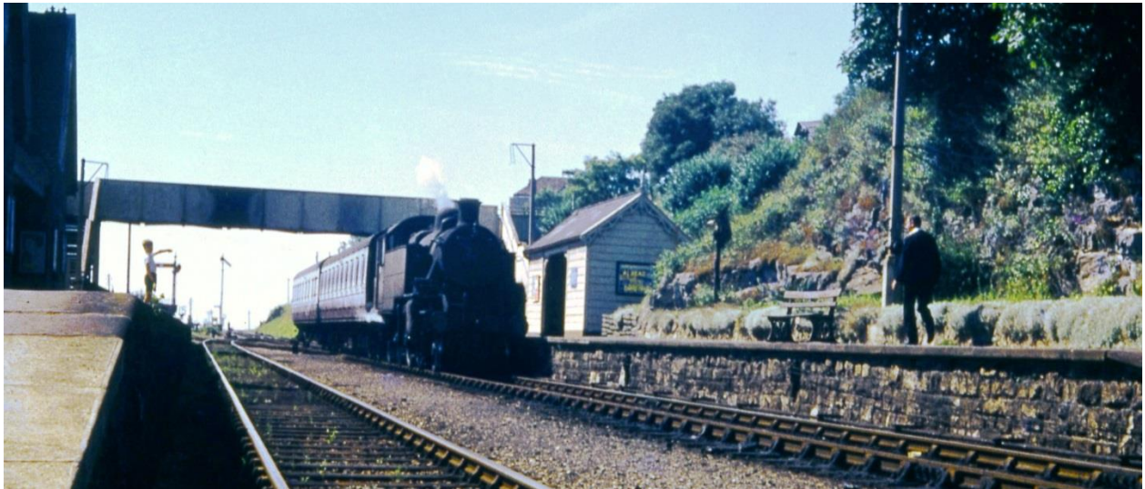
Axbridge station in 1962
