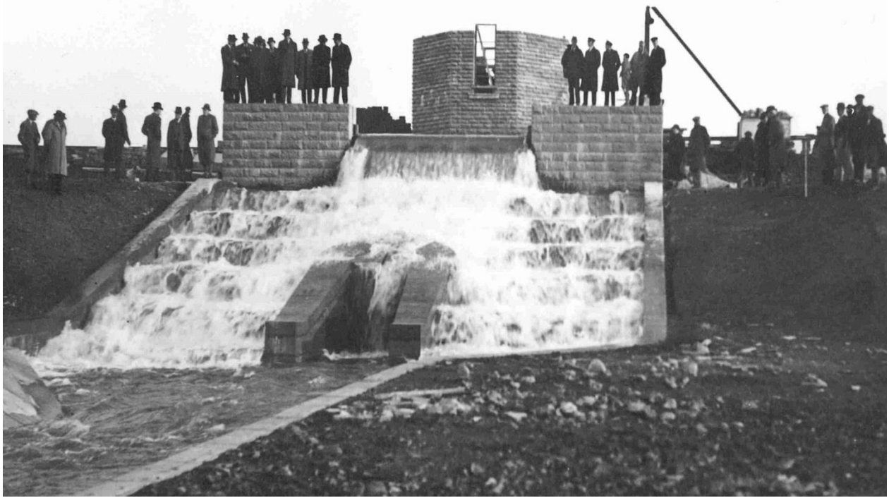
A big moment as water flows in to Cheddar Reservoir for the first time, even though the tower has not yet been completed
