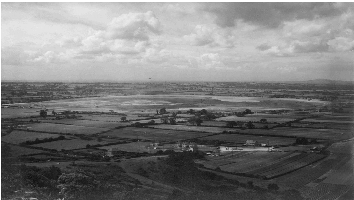
The ground is prepared for the first Cheddar Reservoir
