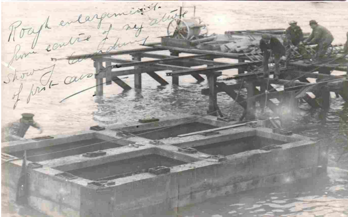
Floating a causeway caisson into position. The photographer penned a note saying this is an enlargement from a wider picture
